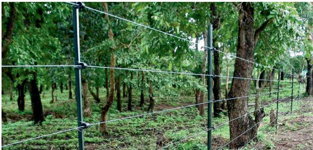
Picture 3: Solar Power Fencing
